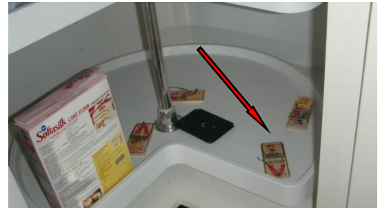
Photo 4INT: Several mouse traps were discovered in various kitchen cabinets. Recommend seal crawlspace exterior vents and clean all food particles from cabinets to mitigate.
