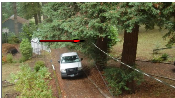
Photo 1ELE: Tree branches should be cut away from wire.
